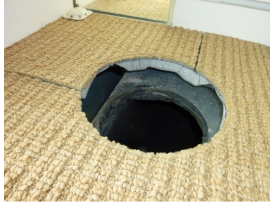
Figure 34: Poorly constructed perimeter diffuser installation
