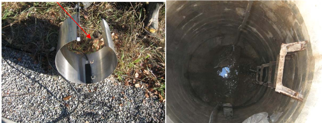
Figure 3: Velocity sensor and its location in manhole
