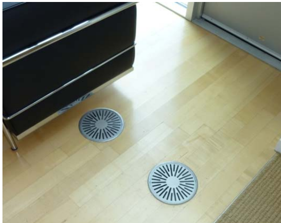
Figure 32: Diffusers placed too close together
