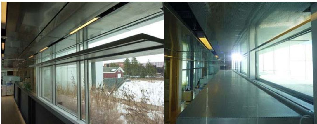
Figure 9: Light fixtures not far enough from the light shelf, resulting in wasted reflected light energy
