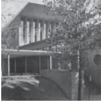
Community Art and Theatre Facility Center of Creative Arts University City, Missouri
