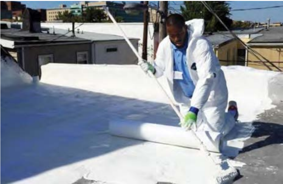
Exhibit 8. Cool roof installation at the Resiliency Hubs pilot. Source: City of Baltimore, 2015.
