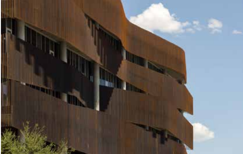
The building exterior is covered in a “blind” that filters direct sunlight. Timmerman Photography
