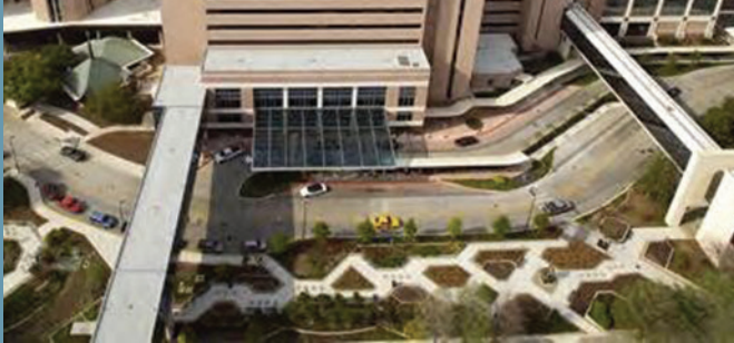
Figure 26: This aerial view of Texas Medical Center illustrates the creation of landscape buffers to enhance stormwater management.
