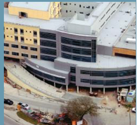
Figure 21: Tampa General Hospital's emergency department is on the second floor, well above the flood surge and inundation level. The vehicular ramp is shown here.
