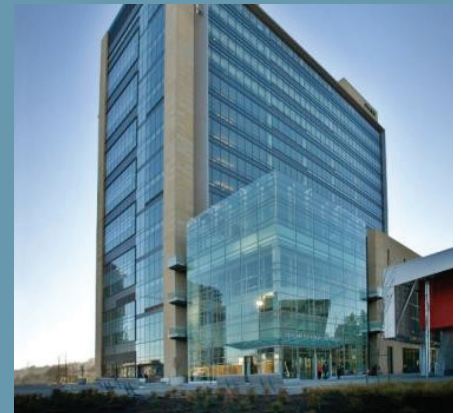
Figure 20: The Oregon Health and Sciences University Center for Health and Healing uses four separate water systems to reduce reliance on both the municipal potable water system and sewage treatment system. It captures, treats, and recycles the building sewage conveyance water using an on-site bio-reactor system.
