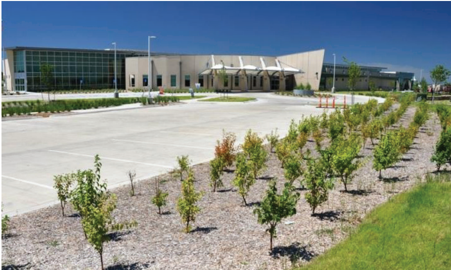
Figure 25: These bioswales at Kiowa County Memorial Hospital filter stormwater and support the Ogallala Aquifer recharge. Rooftop rainwater is collected for irrigation and toilet flushing.
