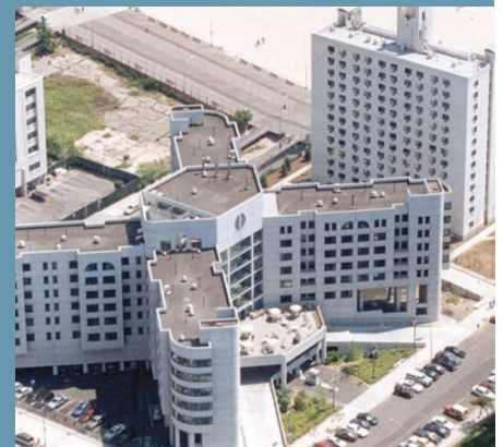
Figure 14: Shorefront Rehabilitation Center, Brooklyn, NY, functioned as planned during and after Superstorm Sandy. The structure was designed to accommodate storm surge at its base levels; all critical infrastructure is above flood elevations.
