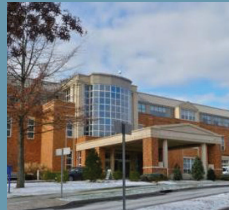
Figure 18: The Greenwich Hospital's on-site combined heat and power system operated without incident throughout the 7-day loss of utility services following Superstorm Sandy.
