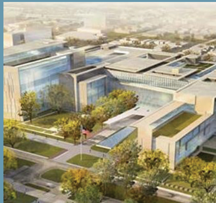
Figure 24: The new Southeast Louisiana Veterans Health Care Center (SLVHCS) features a range of enhanced resilience and infrastructure planning measures. The building is designed to operate for a minimum of seven days, even if all of New Orleans’s utility and infrastructure services are lost.
