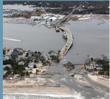
Figure 23: This washed out bridge along the New Jersey shore following Superstorm Sandy demonstrates how vulnerable residential shoreline communities can become disconnected from transportation infrastructure; if large numbers of medical personnel live in such communities, hospitals and long term care facilities must plan to relocate those staff prior to major storm events.
