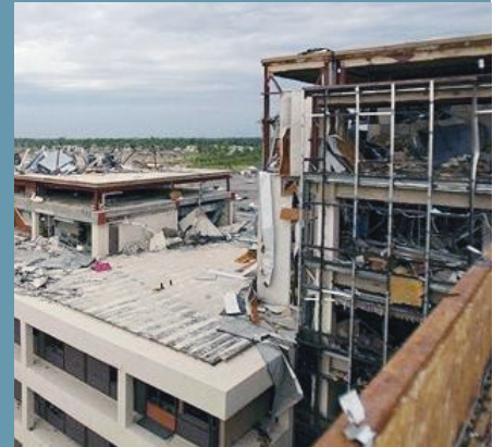
Figure 5: A photo taken from the roof of Mercy Hospital conveys the scope of the devastation. The hospital was a complete loss.
