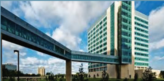
Figure 28: Texas Medical Center improvements include elevated walkways that provide utility distribution as well as advanced stormwater management strategies.
