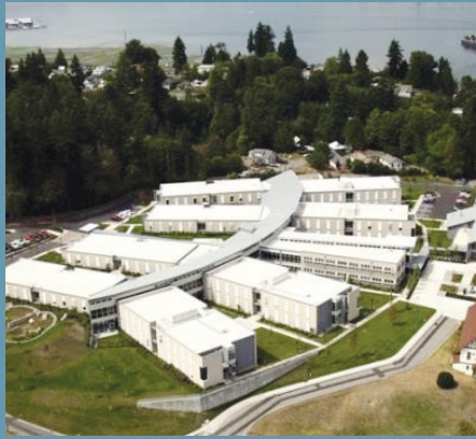
Figure 17: Washington State Veterans' Home orients resident wings to maximize passive cooling and prevailing winds, and includes engineered natural ventilation to replace air conditioning.
